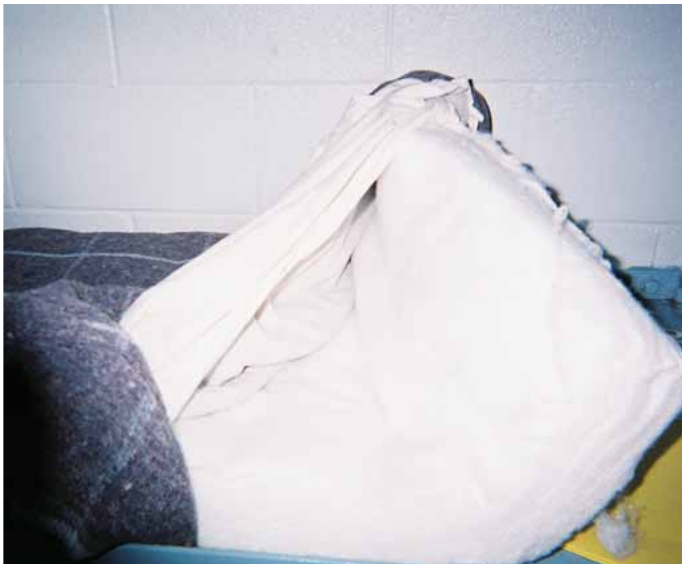
Clogged lint-trap under the only operational dryer on campus (for nearly 200 youth) creating another fire hazard
