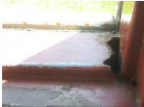
Metal Window Frame
